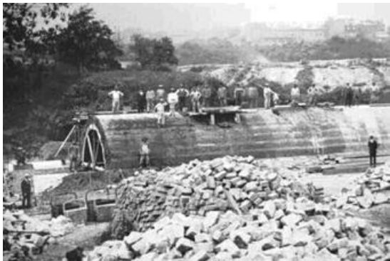
Wingohocking Creek Combined Sewer under construction, 1909
